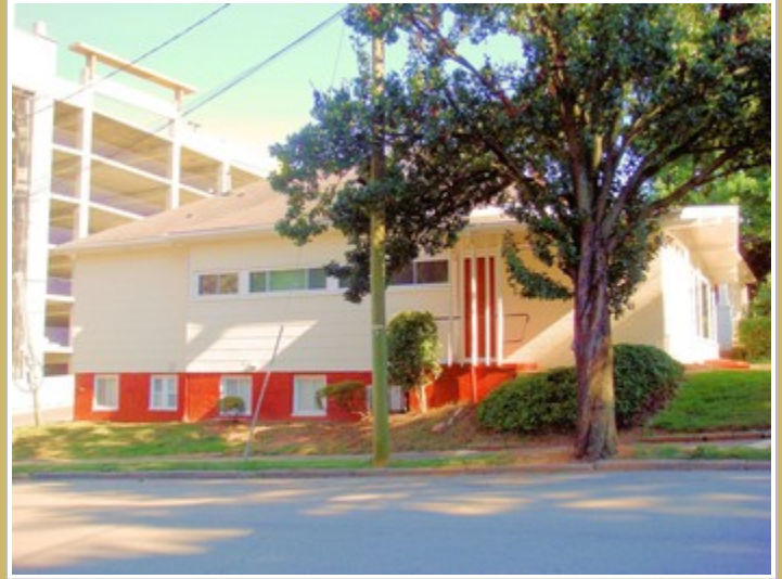
Side View Of Building With Off Street Park
