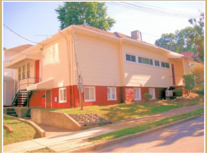
View of Rear Corner and Side Of Building
