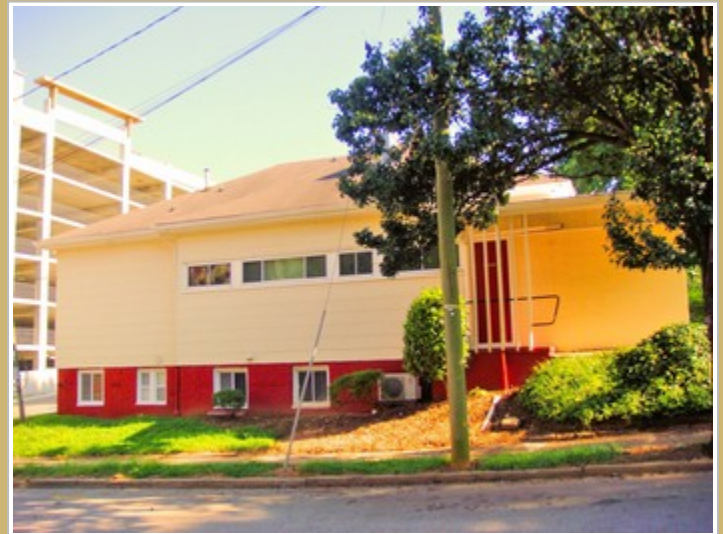
Side View Of Building From Tucker Street
